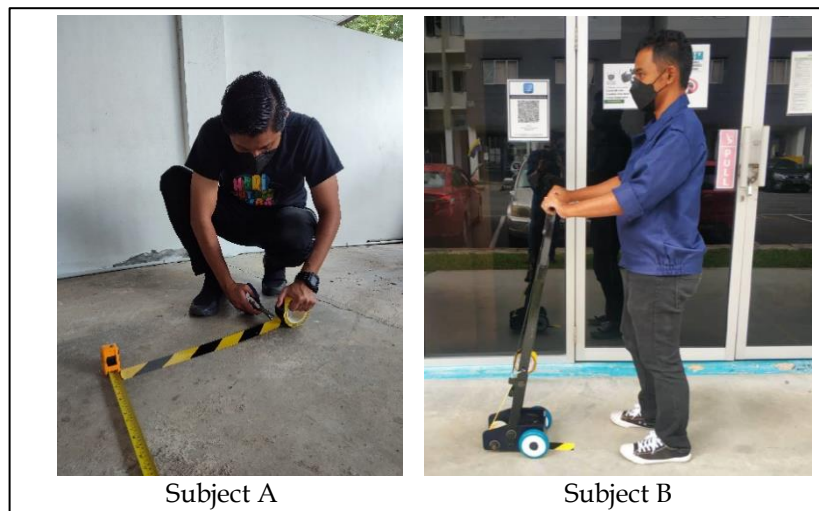
Figure 5. The subjects used different methods to install the safety tape.
