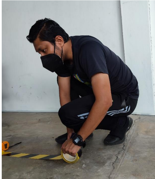
Figure 2. A worker is installing safety tape on the floor.
