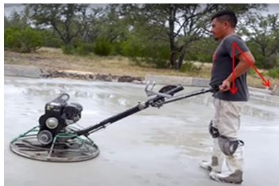
Figure 1: Concrete Trowelling Process Operators
