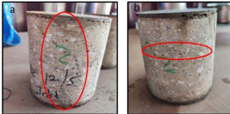
Figure 7: (a) satisfactory failure with crack parallel to the force applied; (b) unsatisfactory failure with tensile crack.
