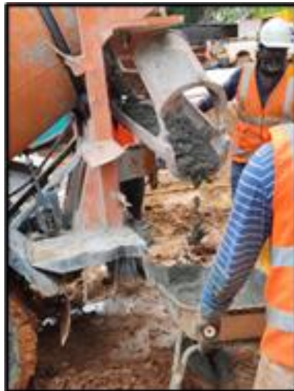
Figure 4: Sampling of fresh concrete for slump testing and cube making.
