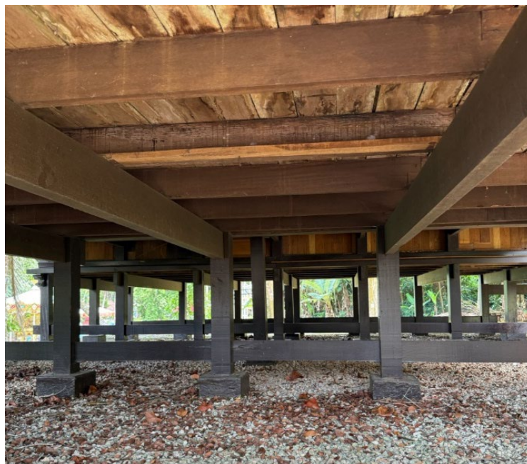
Figure 2: An example of tanggap in a traditional Malay house. Field documentation photographs by the author (2025).
